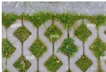
Figure 4.1 Cement grille of eco-friendly city parking lot with green grass
