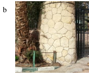
Figure 6.12 (b) : shows the using of limestone in the cladding of the wall
