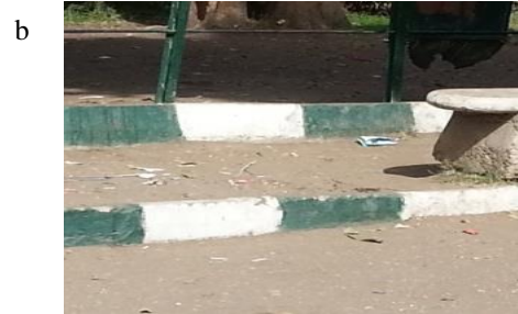
Figure 6.8 : shows the using of concrete in the steps of the sidewalk.
