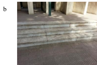
Figure 6.10 (b) : shows the using of the white marble in the entrance stairs
