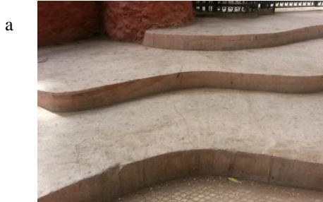
Figure 6.7 : shows the using of concrete in a smooth shape in some places
