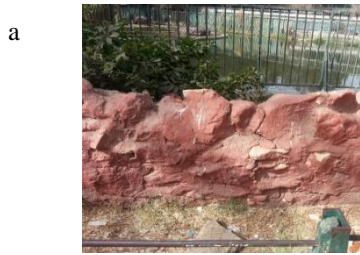
Figure 6.11 (a) : shows the using of the painted limestone Rocks to build a boundary wall for the animals area
