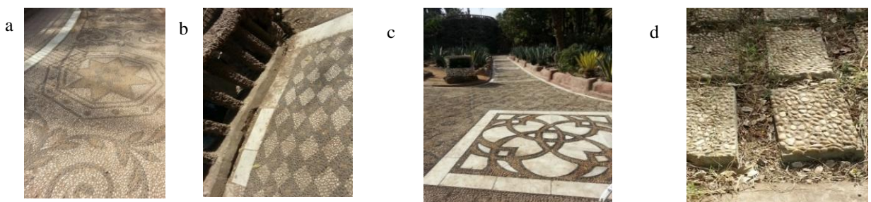
Figure 6.4 (a,b) : shows the application of stone ( specially colored pebbles) in a decorative paving in different shapes and Motifs
