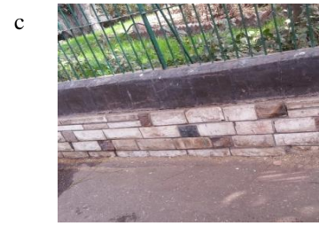
Figure 6.13 (c) : shows the using of the pharaonic stone in the cladding of the wall
