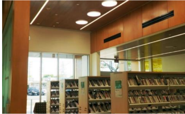
Figure 17 Solatube at South Whittier Public Library.
