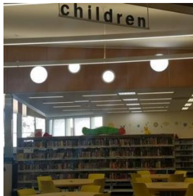
Figure 18 Installation of solar tubes in the ceiling above the bookshelves. This will allow the evenness of natural light throughout the space via the transparent lighting tubes.
