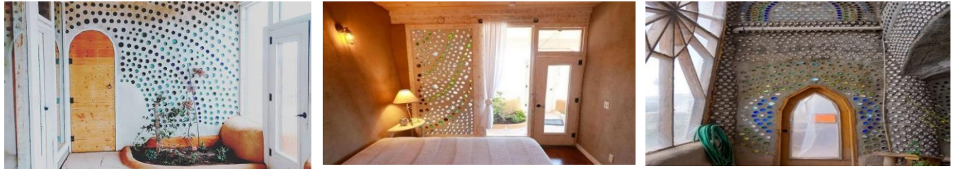
Figure 11. Recycled Bottles and Cans Create a Stained-Glass Effect [29,30].
