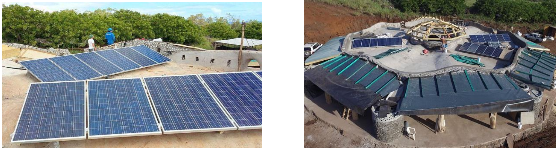
Figure 16. Set Solar Panels on the School's Roof [32]
