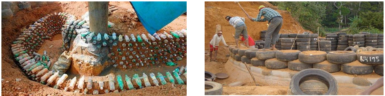
Figure 4. Construction using Tires, and Plastic Bottles [17].
